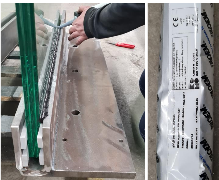
Image 14 Sealing the glazing using EASYSEAL XPS®
