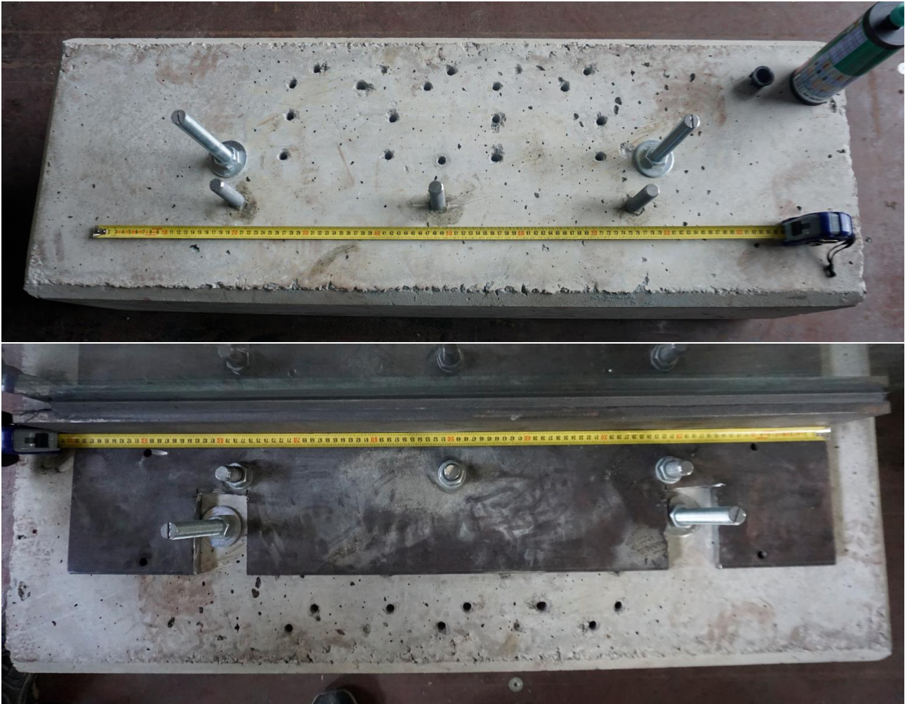
Image 5 Mounting of the substructure
