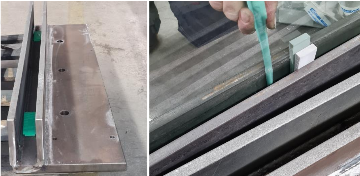
Image 12 Glazing blocks and injection point of the adhesive
